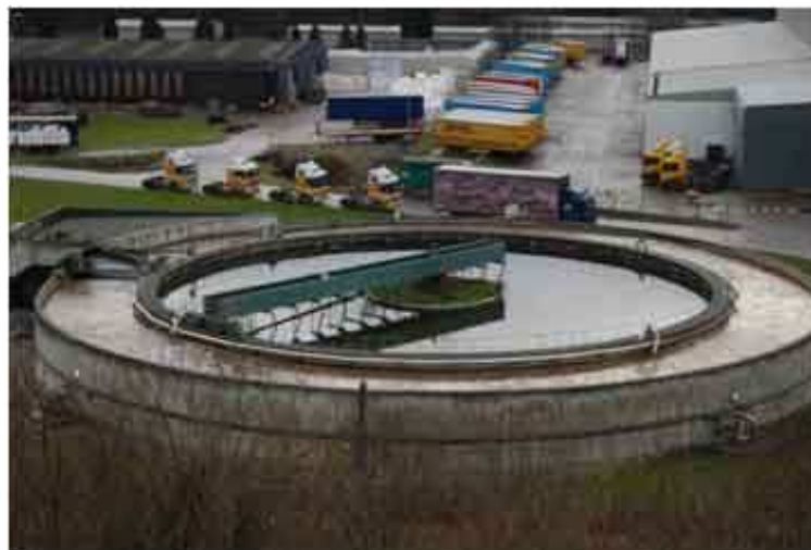
Figure 14.22 - a water waste treatment 31 plant
