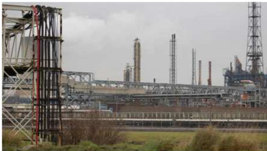
Figure 14.31 - an industrial chemical plant
