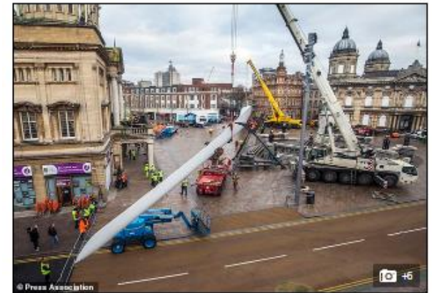
The pieces was moved into place
