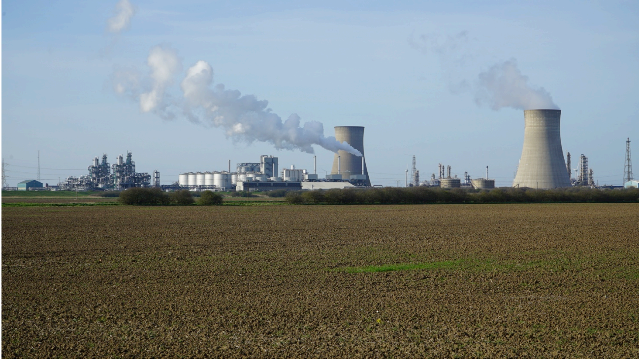
LOCATION: chemical plant in distance 1
