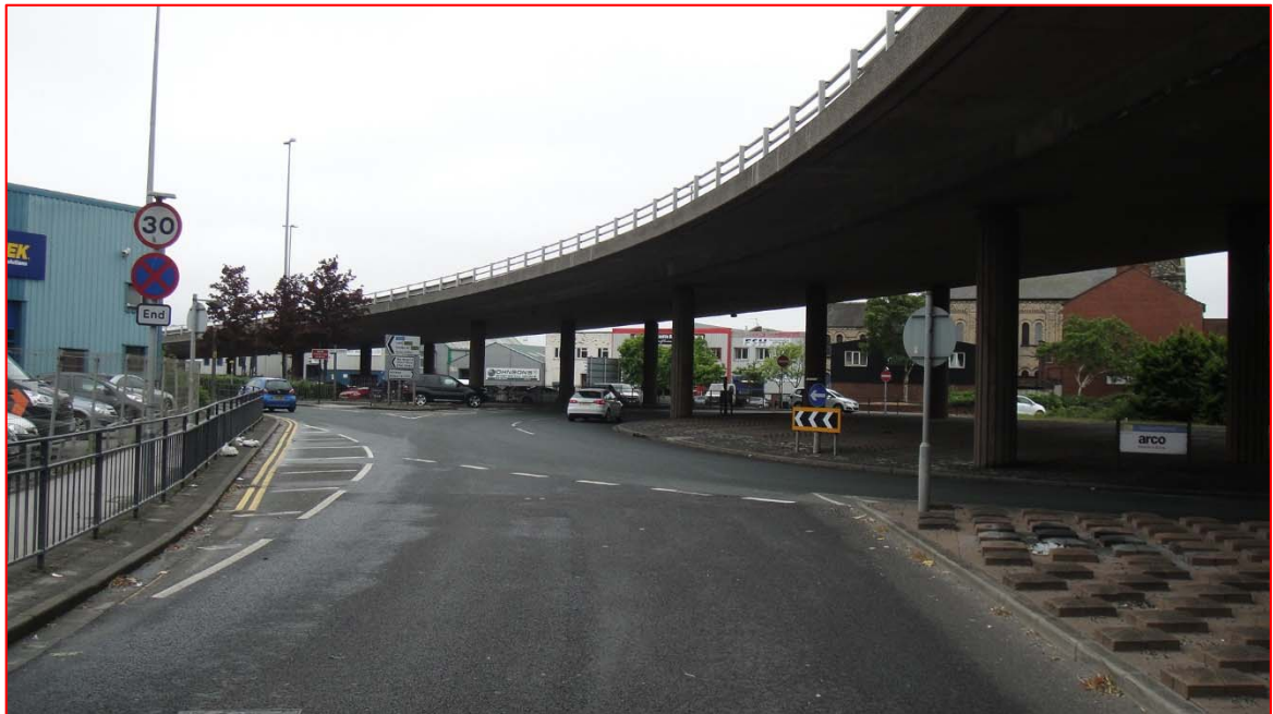
Photo Reference 7 - Bridge height 5.4 metres above road surface - height restriction
