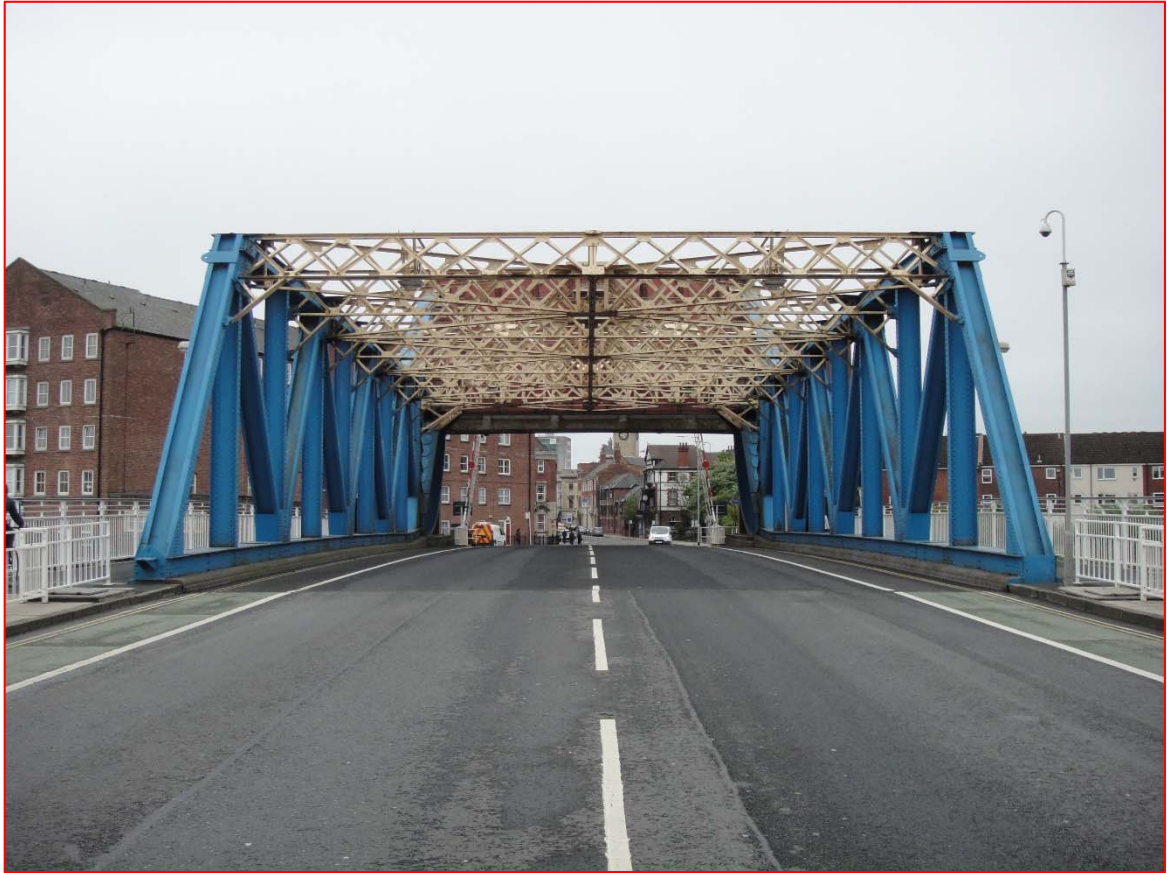
Photo Reference 6 - Bridge height 5.85 metres above road surface – height restriction
