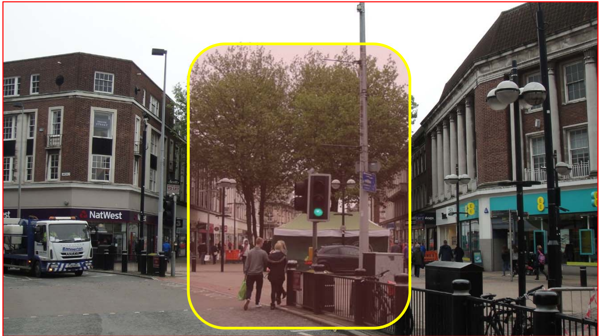
Photo Reference 18 – junction of King Edward Street and Jameson Street. Proceed through pedestrianised area to King Edward Street. Street furniture to be removed. Note trees. Potential tree surgery to be carried out.
