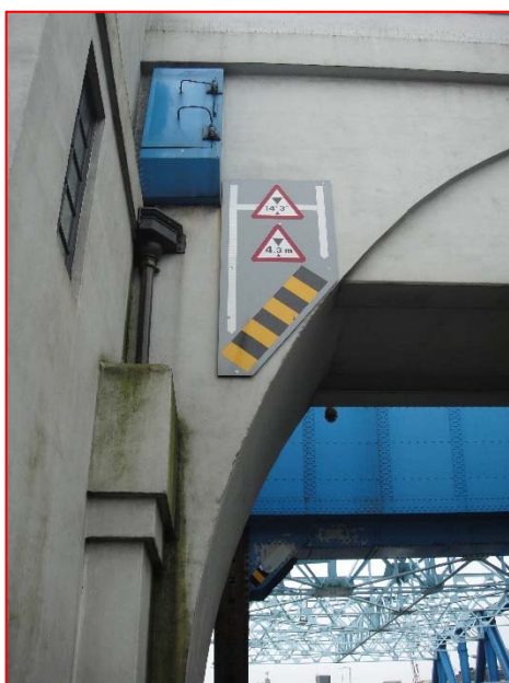
Photo Reference 5 – Bridge height 4.3 metres (14'-3") above road surface – height restriction
