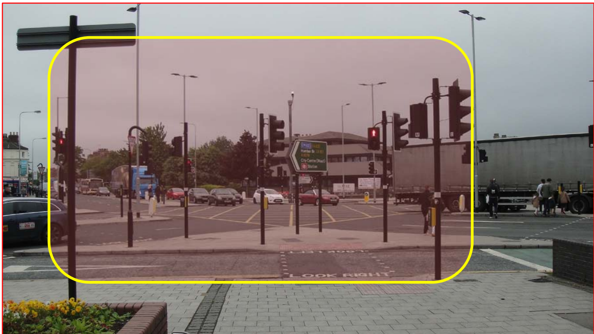
Photo Reference 14 – junction of Ferensway with Prospect Street. View looking from Prospect Street – all street furniture to be removed from central part of intersection of both roads
