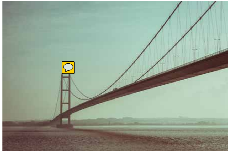
287 Humber Bridge Photo: © Chris Pepper
